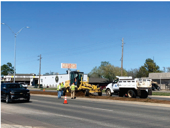
Hwy 81 Medians re-graded to ensure safety of crews during maintenance work.
